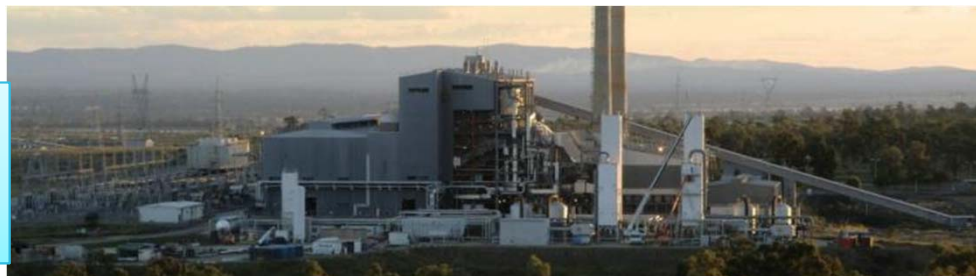
Callide Oxyfuel Project
